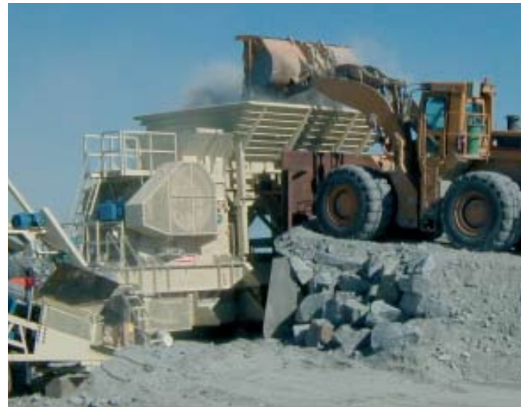
Mobile crushing with the NW125.
