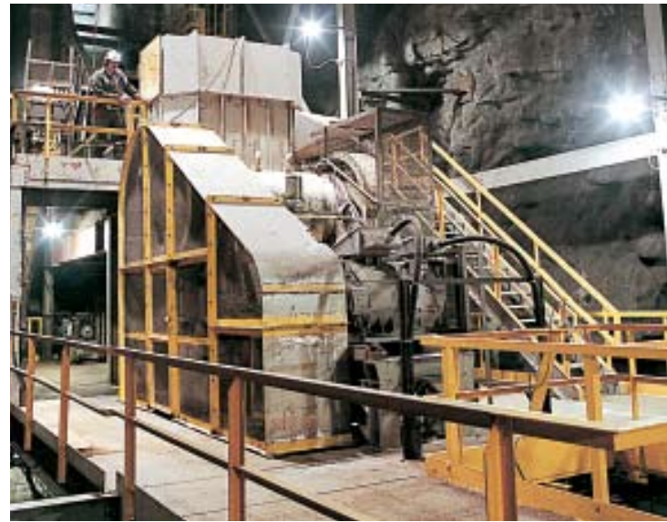
C160 at an underground gold mine.
